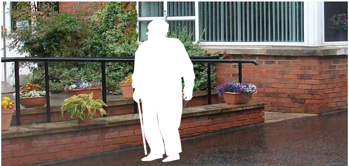
12 Steel handrails to exterior ramp.
