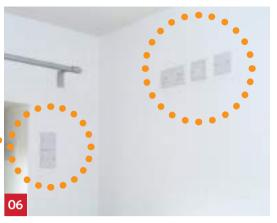
Data and power connections are provided at 2300mm for future assisted living technologies installations, and adjacent to windows for actuators.
