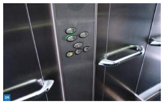
Inside lift with handrails, mirrored surface at correct heights and large numbers with Braille on the buttons. The lift buttons shown in the photo should contrast more with the surrounding lift wall to make them easier to see.
