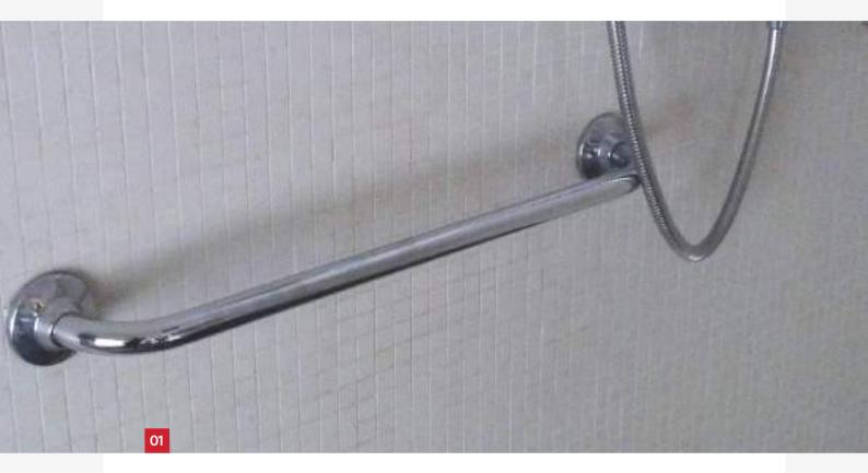
A strong load bearing surface has been provided throughout the shower room to allow for firm fixing of handrails wherever they might be required.
