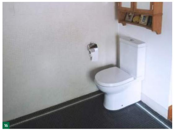
Good large clear space in front and to the side of WC. Storage provided within bathroom. Colour contrast between the WC and wall should be greater to make it easy to find for everyone.
