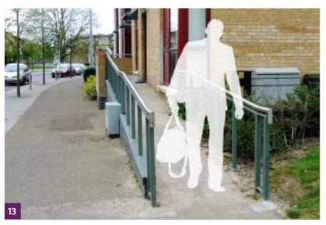
Ramp and landings provided to raised ground floor with handrails on both sides.
