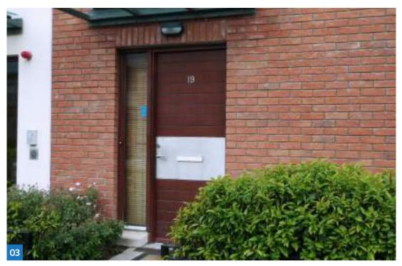
A glazed panel beside the door gives daylight to the hallway and views in and out. The door furniture is at an accessible height, the number is clear, and a light is provided. There is good contrast between the brickwork and the door.
