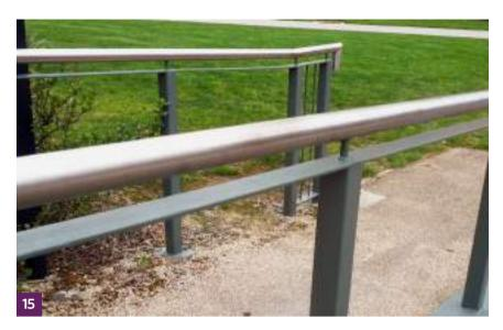
Handrails provided on both sides of ramp, and following the line of the ground surface. Supports do not get in the way of hands and the railing turns downwards at the end to avoid clothes getting snagged.
