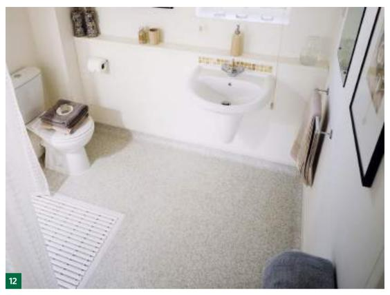
The level access shower has a recessed drainage area and the basin can be used by someone seated. Ideally there should be better colour contrasts.
